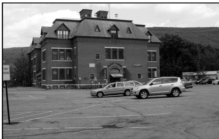
Brattleboro Municipal Center today, hockey area is a parking lot. Annex was removed long ago to make room for more parking. (Photo: Lee Ha, 2013)
