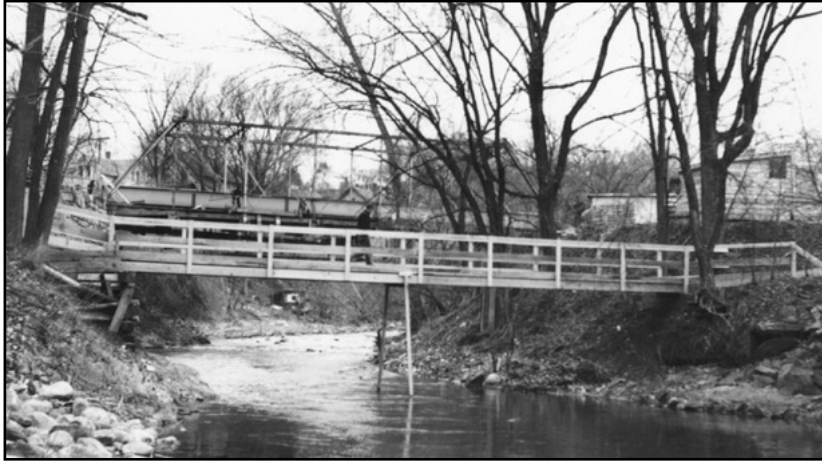
Photo above: Elliot Street Truss Bridge being dismantled in the background and a temporary foot bridge in the foreground, across the Whetstone Brook. (BHS Photo Collection, 1948)
