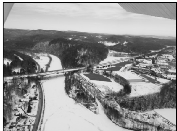
In the Fall of 2013, the I-91 West River Bridge reconstruction began and by January 2017, though nearing completion, it was not yet drivable. Facing West. (BHS Photo Collection: Joseph Yudin, 2017)
