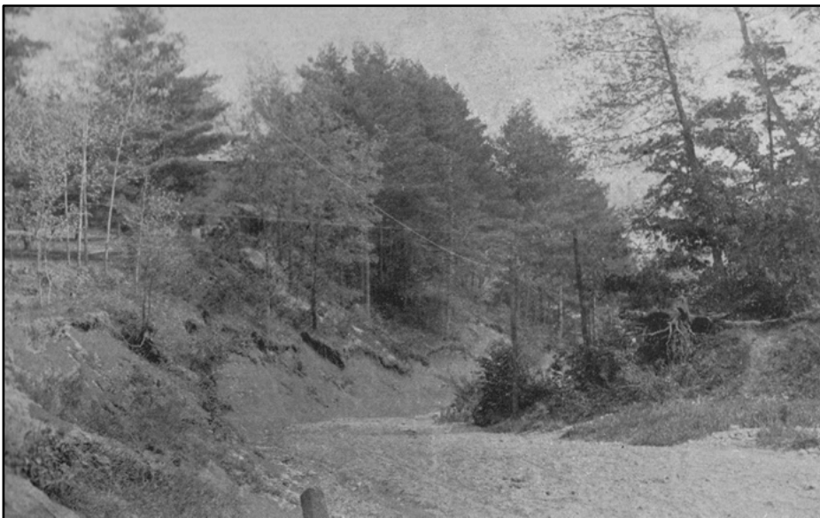
From Western Avenue facing south. This picture shows Union Street about 10 years after it was laid. Notice the embankment and depth of land taken to make the grade of the road passable. It now becomes obvious why the top of Union Street was so wide, to be navigable for teams of horses and freight. Modern times have proved this dangerous for pedestrians and Union Street has recently been made much narrower at the top. (Picturesque Brattleboro, 1896)
