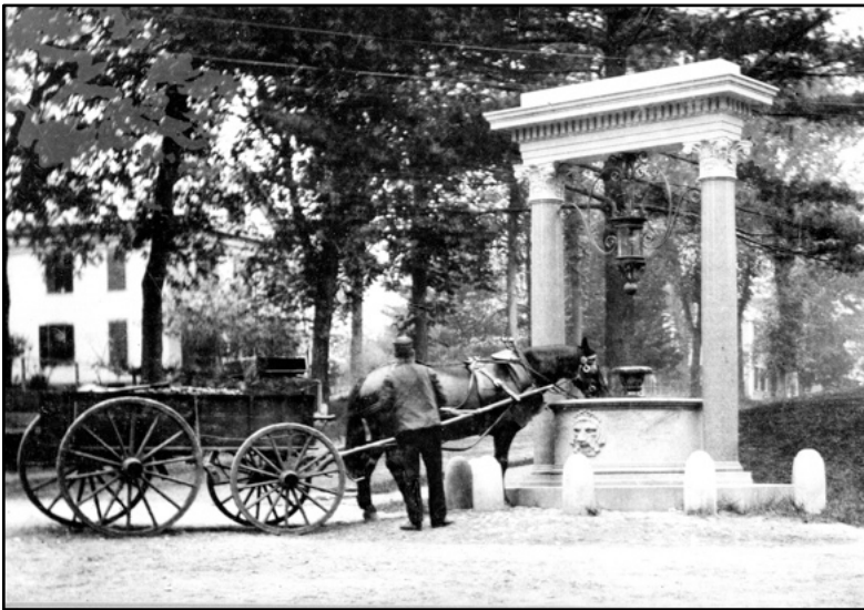
Surrounding one of Brattleboro's landmarks, bollards were placed to help protect the new Wells Fountain in 1890 at the intersection of Linden Street (then Asylum Street) and Putney Road. Nearly 100 years later, in 1989, Wells Fountain was moved farther up the hill, the bollards were removed and thankfully saved. (Photo: BHS Photo Collection, c. 1890)
