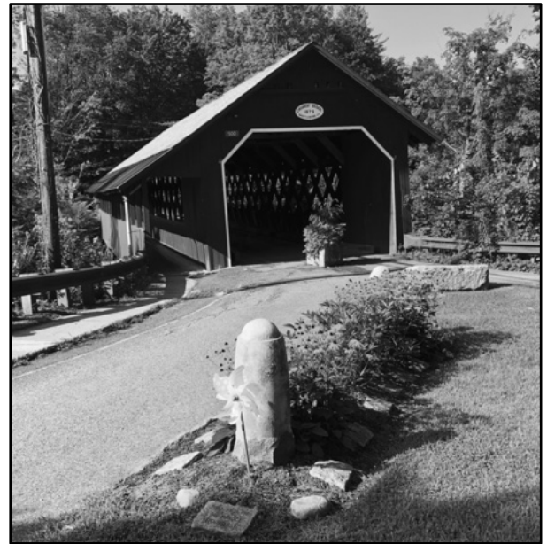
When the Citizens Bridge was built and the Creamery Bridge became a foot bridge, four of the bollards were added to enhance two beautiful well-tended gardens. One bollard is visible above. (Photos: Lee Ha, 2018)
