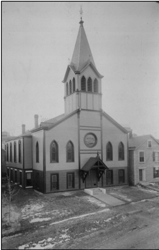
Universalist Church, Canal Street, note stained glass circular window (Photo: BHS Photo Collection, c. 1890)
