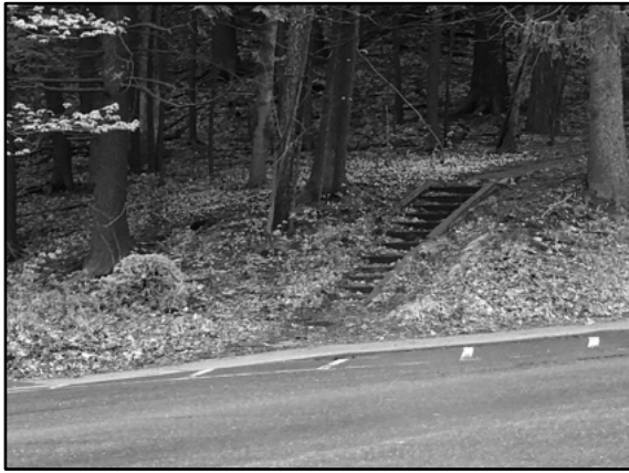
Derelict stairs leading into the woods at the corner of Pine Street and Maple Street. (Lee Ha, 2019)
