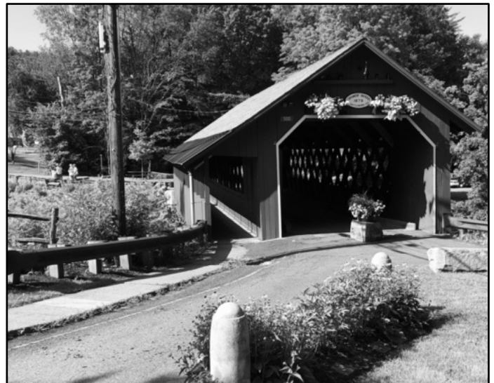
Creamery Bridge, built in 1879, is no longer used for traffic. Note the added walk on the east side of bridge. (Lee Ha, 2019)
