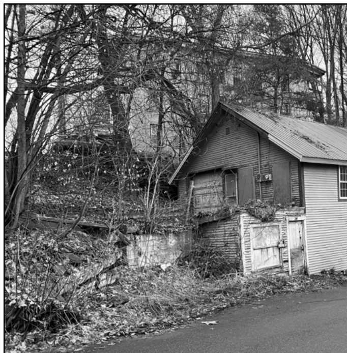
Now: Notice the deteriorating retaining wall which is now overgrown with both weeds and small trees. Also note the apartment building in background, the original Methodist Church. (Photo: Lee Ha, 2019)
