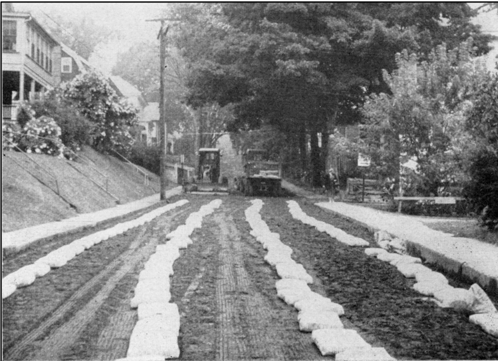
Distributing cement on Grove Street soil-cement project
