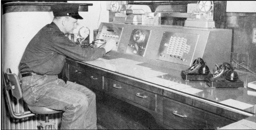
1949: The Central Station fire alarm equipment. "...the instrument that transmits box alarm signals to the audible alarm mechanism. Telephone alarm calls are also set up on this instrument for transmission." This new equipment was supplied by the Superior American Fire Alarm and Signal Company at a cost of $13,300. (Lewis R. Brown, 1949)
