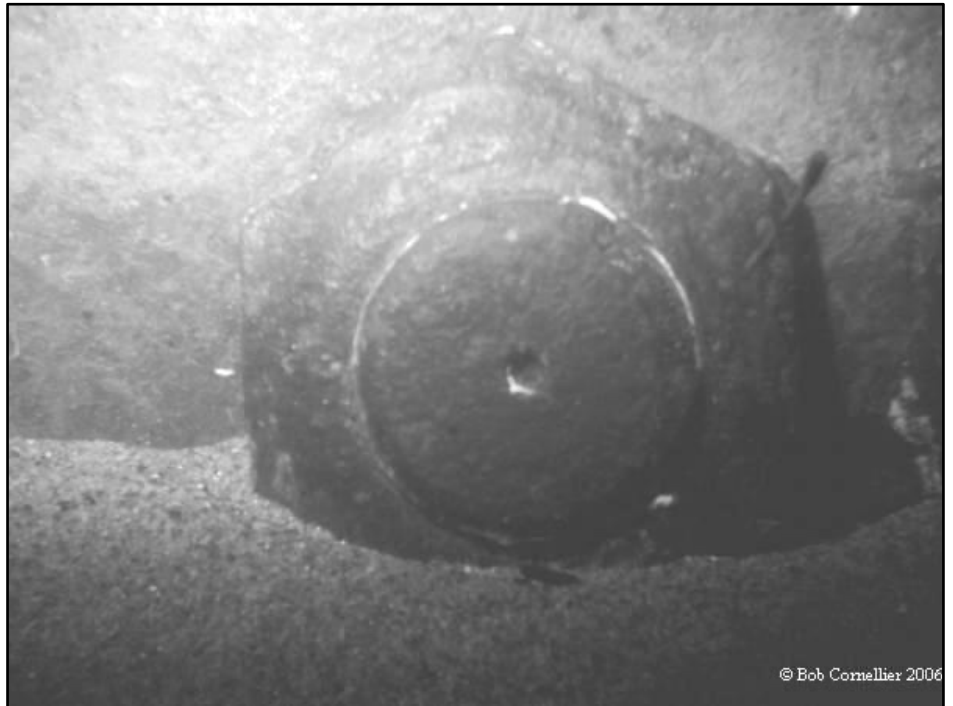
Part of the bridge washed out in 1929. (Photo: Robert Cornellier, 2006)
