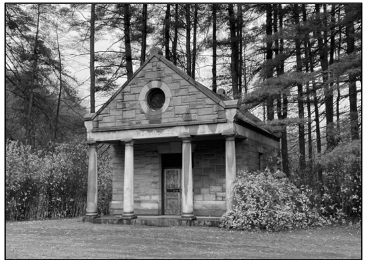
Morningside Mausoleum. No longer used, a solid building showing its age. All windows, including the circular window, are now boarded up, a large padlock secures the door and it's surrounded on 3 sides by overgrowth, with a backdrop of stately white pines. (Lee Ha, 2020)
