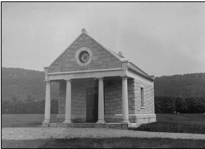
Morningside receiving tomb and chapel built in 1900 is 24 x 31 feet and built of Dummerston granite with a large porch and pillars of the same. The interior is finished with white marble and white enameled brick and windows are stained glass. (BHS Photo Collection, 1900)
