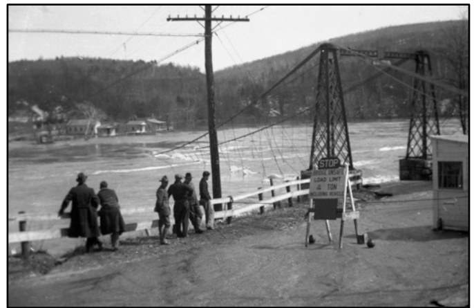
The suspension bridge collapsed into a raging river during the flood of 1936. Notice the difference in the width of the Connecticut River from the photo to the left. (BHS McVeigh photo collection, 1936)
