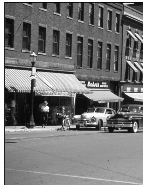
East side of Main Street hill with the building that was of Goodnow, Pearson & Hunt. The building is part of the American Building.
