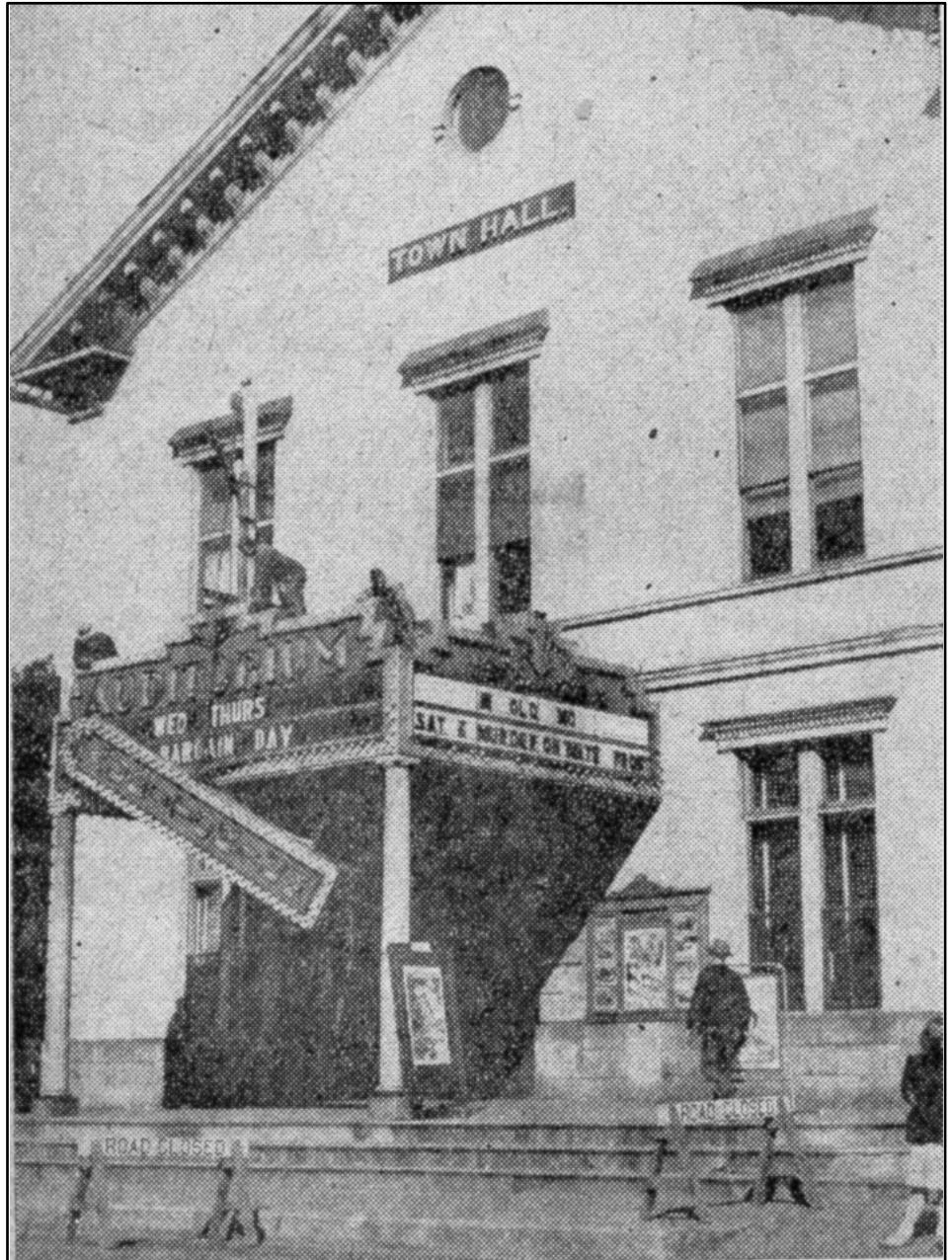
Water department employees lower first piece of auditorium marquee to ground as removal gets under way. (Brattleboro Reformer, October 7, 1943)
