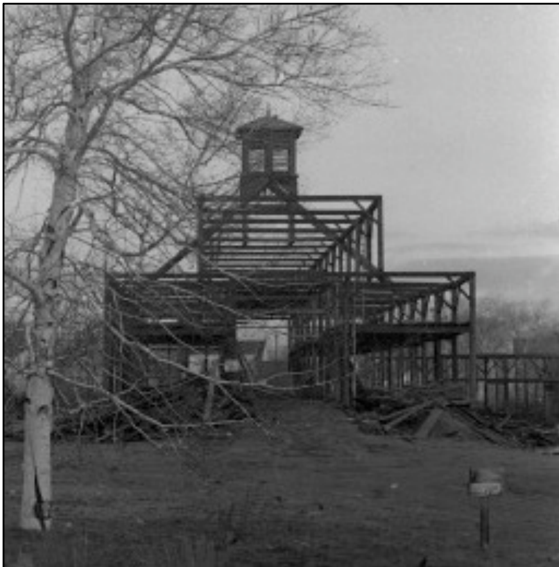
John D. Latchis barn being dismantled on Fairview Street, at the acurrent location of HCRS Health Care/Rehab Services. This property was previously owned by Henry G. Clark, his farm encompassed many acres on Canal Street, now the Market 32 complex. As the barn was dismantled, the highly sought after barn board was sold. (BHS Brattleboro Reformer Photo Collection, 1969)
