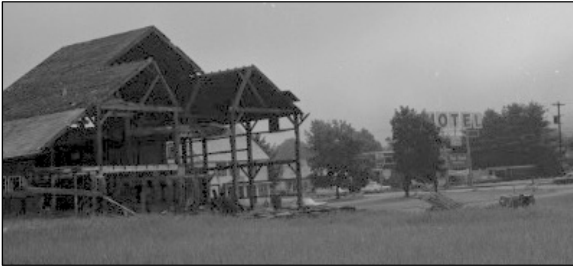
The Thomas Farm, demolished in 1978. The majority of the property on the west side of Putney Road encompassed the vast George Thomas Farm. (current location of Hannaford Plaza). After the initial demolition, the fire department used the remaining building debris for a training fire. (BHS Brattleboro Reformer Photo Collection, 1978)
