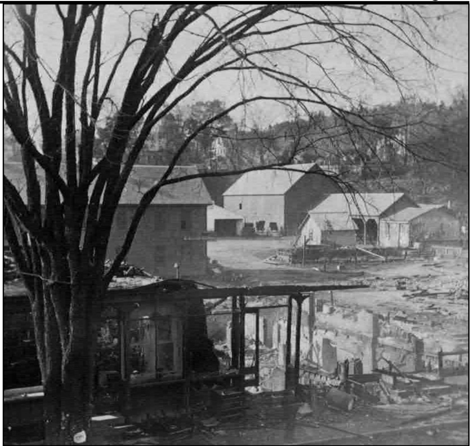
Above: Elm tree damaged by the huge fire in Brattleboro which burned the entire west side of Main Street between High and Elliot Streets. (BHS Stereocard Collection, 1869)
